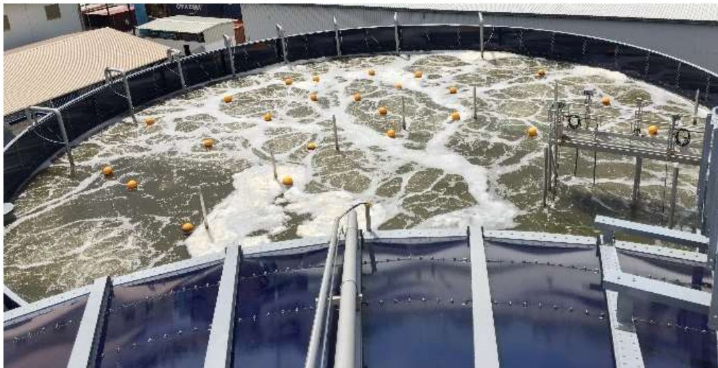
Aeration tank and MBR modules
